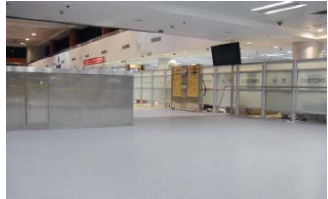
香港罗湖站航站楼 HK Lo Wu Station Terminal Building ARDEX CL 11, ARDEX P 51, ARDEX WPM 300
