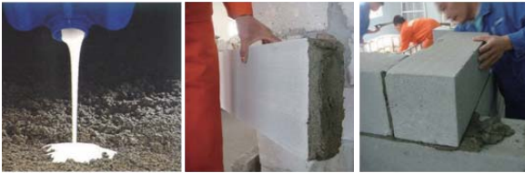
(2) 粘接力强，堆头不掉浆，干法砌砖
